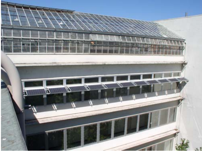
Fig. 1: Solar awning on the third floor of Pacific Hall. The modules are separated into two strings of six to minimize the shading problem on the whole system. The hallway on the second floor will be used as a control.
